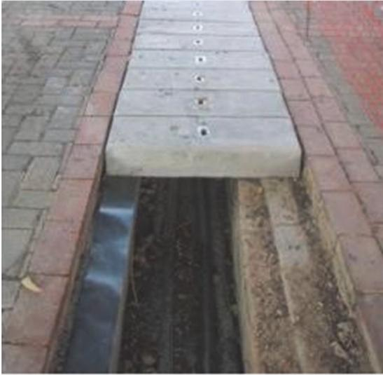
Figure 4: UG Cables with Concrete Channels - II
