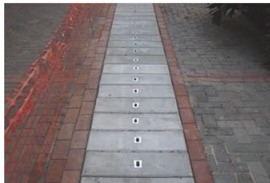
Figure 3: UG Cables with Concrete Channels - I
