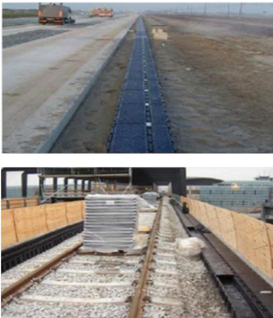
Figure 7: MultiRex cable Channel Installations
